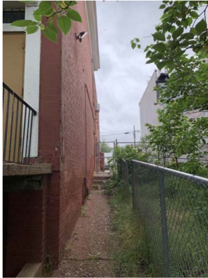
EAST SIDE YARD
